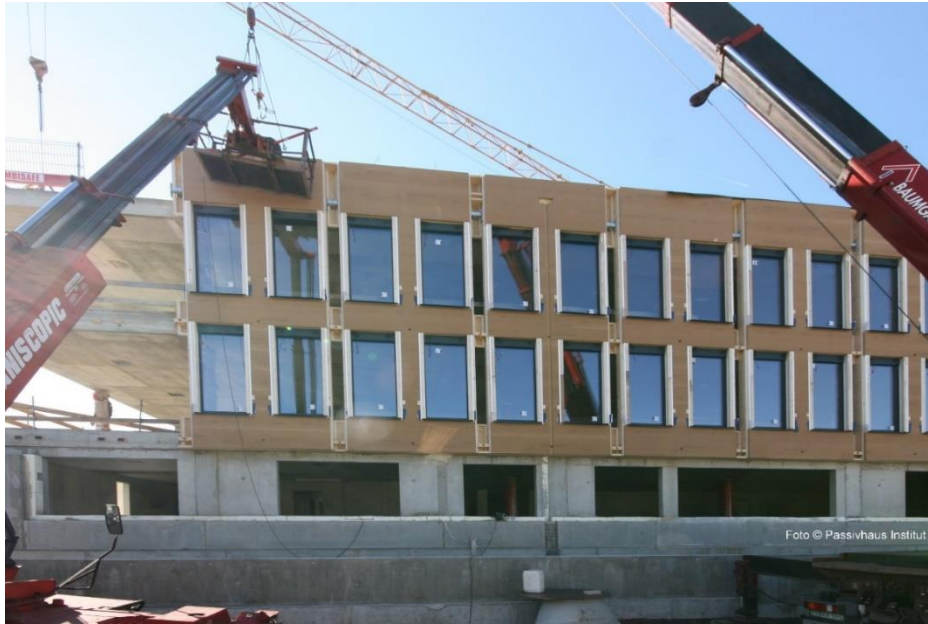
Fig. 4: Assembly of the prefabricated façade elements
